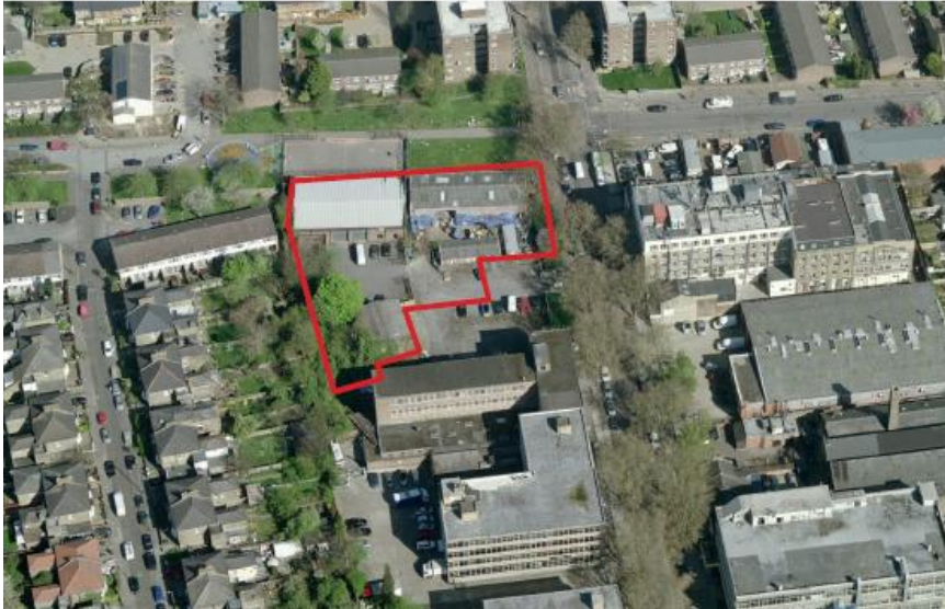
Aerial view – 45-63 Lawrence Road
